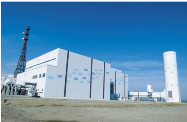
Ishikari Bay New Port Power Station (LNG thermal power station) (source: Hokkaido Electric Power Co., Inc.)
