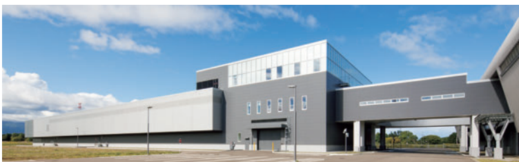
Ishikari Data Center Building 3, built by SAKURA Internet Inc. in Ishikari City in December 2016
